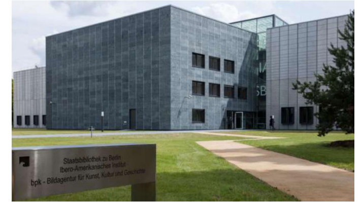
Storage facility Friedrichshagen (SE of Berlin) (2014)
